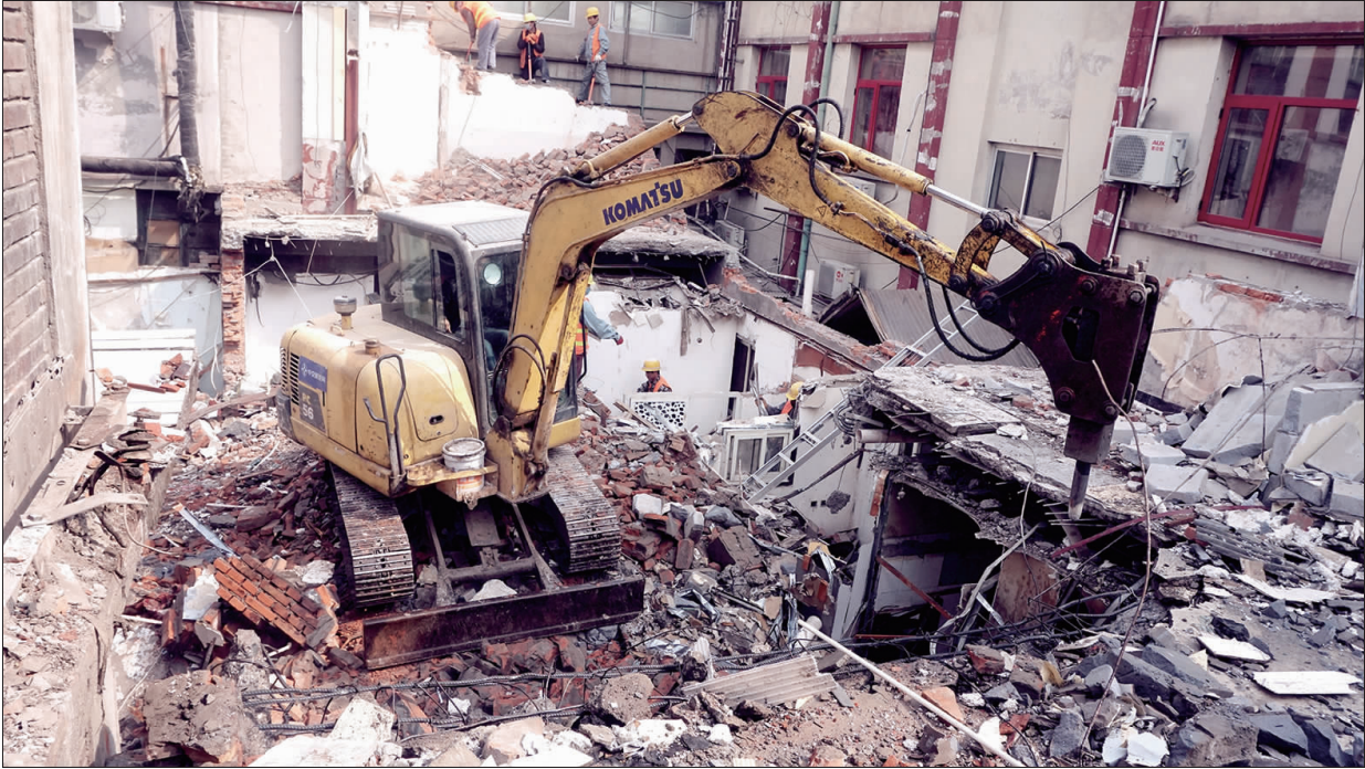
拆除饶丰宾馆违建
